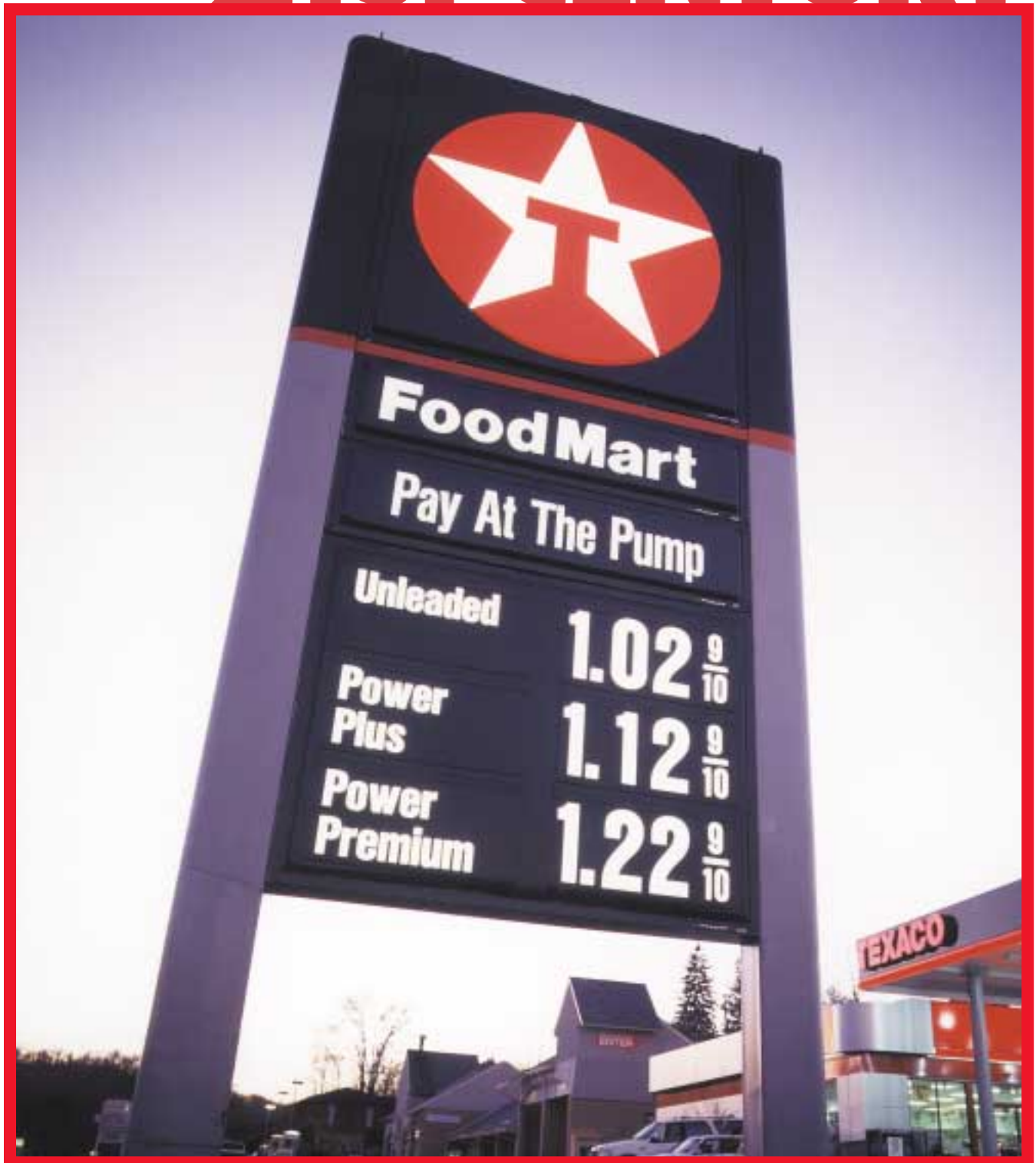
D-shaped HSS sign support columns provide improved durability and cost savings.
